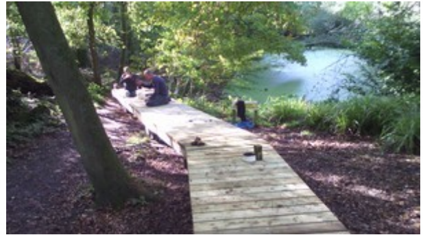
New Boardwalk under construction. Picture; Tony Morton
